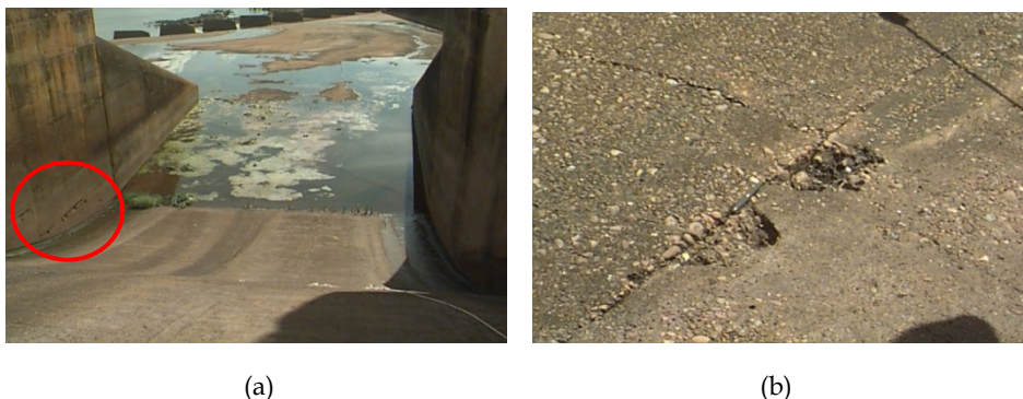
Fig. 2. (a) Spillway dam presented deterioration by abrasion. (b) Defects in the concrete structure caused by abrasive process
